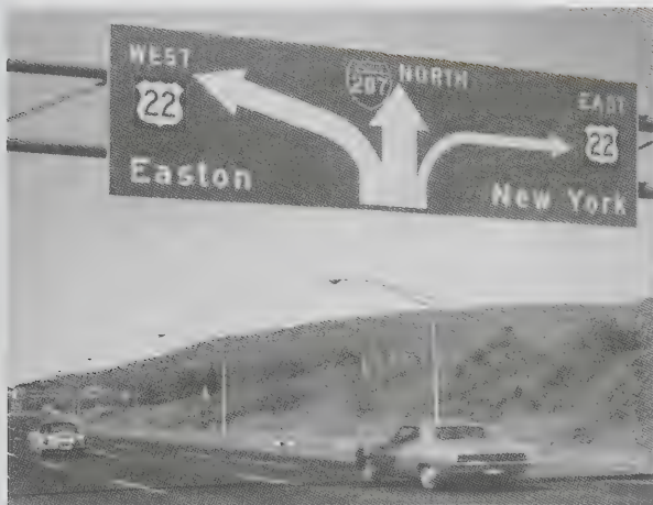
Diagrammatic traffic signs installed at the I-287 and Route 22 interchange – the first such signs used in New Jersey. (1969)
